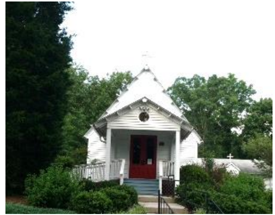
St. Andrew's Episcopal Chapel (1906 – 1955) Originally at Green River Plantation, Polk County, Diocese of Western North Carolina Photo: chapel after 1955 relocation in Tryon
