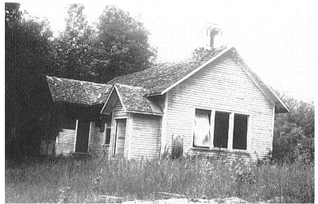
St. Saviour's Episcopal Church (1931-1944) Formerly in Macclesfield, Diocese of North Carolina Photo: Property Survey Records, Diocese of North Carolina c. 1938
