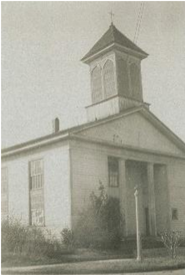
St. Cyprian's Episcopal Church (1903 – Present) 408 Granville St., Oxford, Diocese of North Carolina Photo: 1927 building
